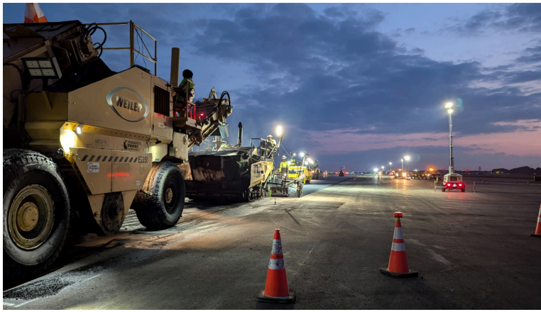
Figure 2. Nighttime paving operation on airport runway
