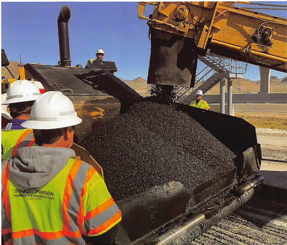
The HiMOD mix's homogenous nature and the depth of the lift milled section in front of the paver. PHOTO COURTESY STAKER PARSON AND ASPHALT PRO
