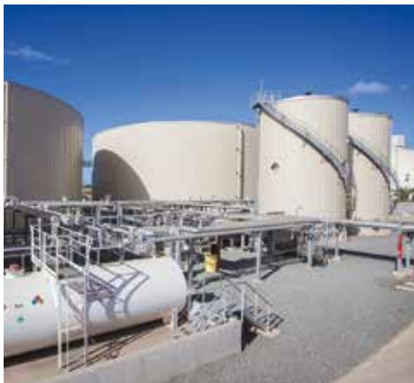
Asphalt Terminal Kalaeloa Harbor.
